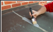
• Protection against corrosion on lead and zinc
