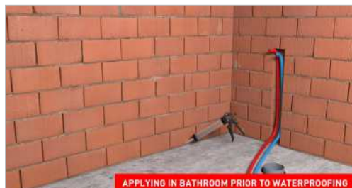
APPLYING IN BATHROOM PRIOR TO WATERPROOFING
