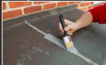
• Protection against corrosion on lead and zinc
