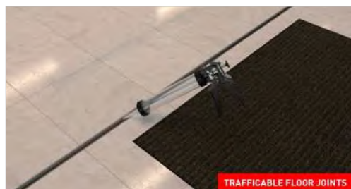
TRAFFICABLE FLOOR JOINTS
