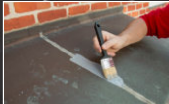
• Protection against corrosion on lead and zinc
