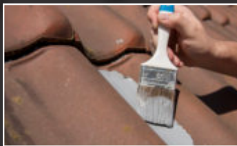
• Roof tiles and -edges
