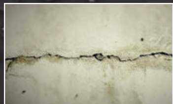
• Concrete foundations and cellars
